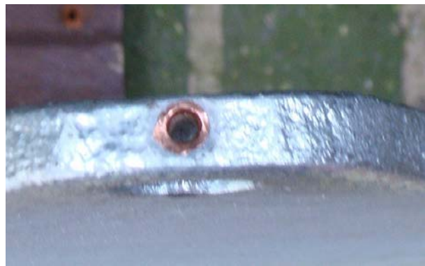
Fig 14: Copper tube hole liner top view
