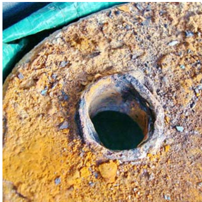
Fig 8: Original bush in place
