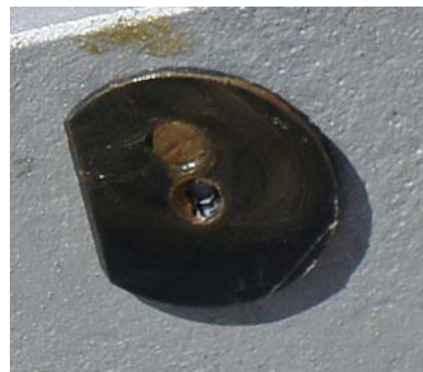
Fig 12: New HDPE pad
