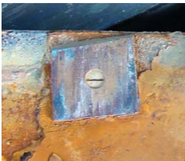
Fig 11: Original Tufnol pad
